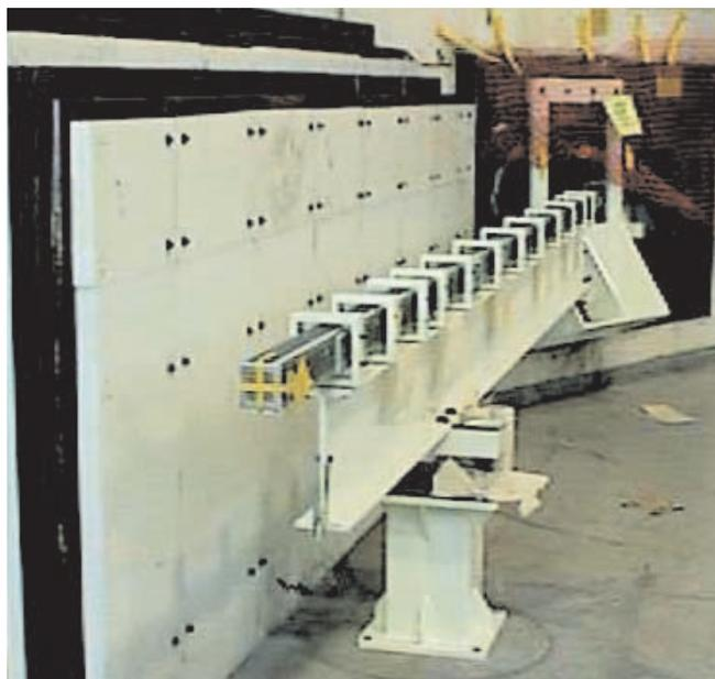
Fig. 2. Neutron guide prior to shielding installation
